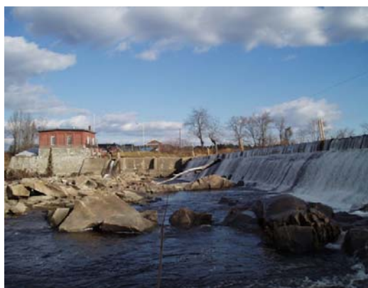
Figure 4.3.1. Before Sandy River Project
