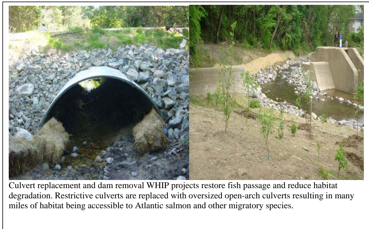
Figure 4.5.4. Example of Culvert Replacement and Dam Removal Projects
