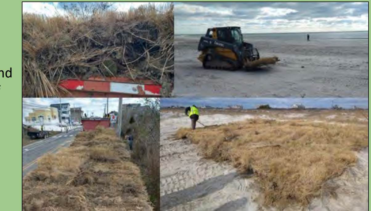
Figure 9: Photos of Strathmere demonstration planting: trailer of conservation plant sod slabs (left), saltmeadow cordgrass slab transported to dune (top right), and sod slab trial plot (bottom right).
