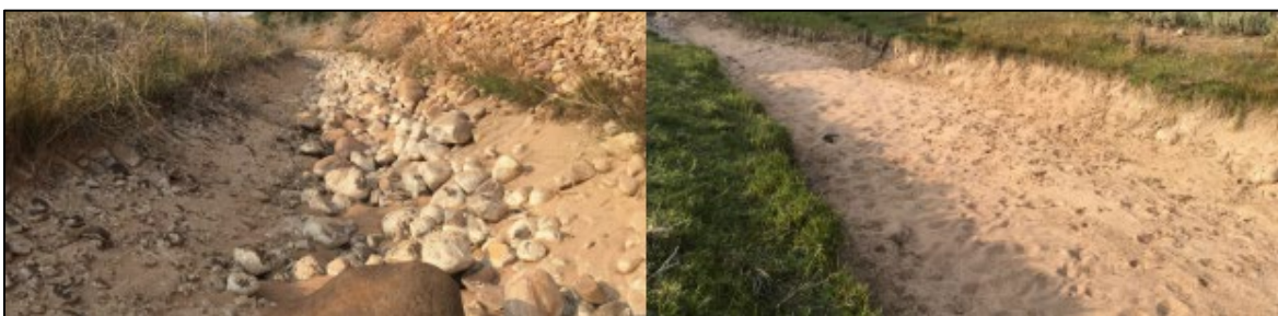
Figure 2-1. Unlined Sections of Yellowstone Feeder Canal
