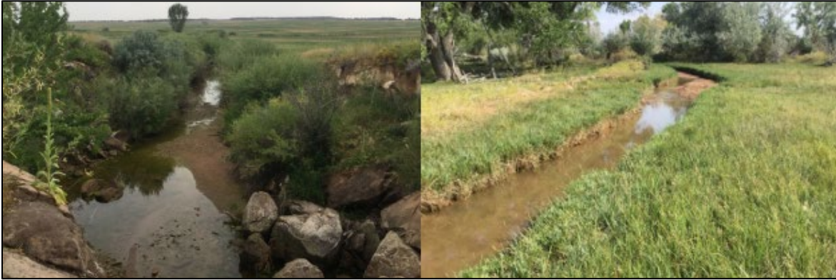
Figure 2-4: Dry Gulch Class B Canal
