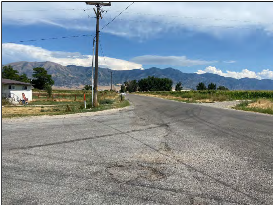
Photo 14: Location in Bear River City where proposed pressure irrigation improvements would occur, looking east.
