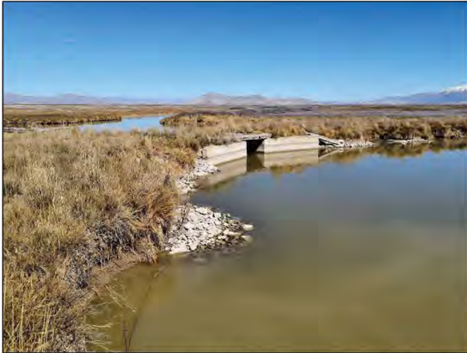
Figure 11. IF-10, isolate overview, headgate in modern concrete channel; view facing northeast.
