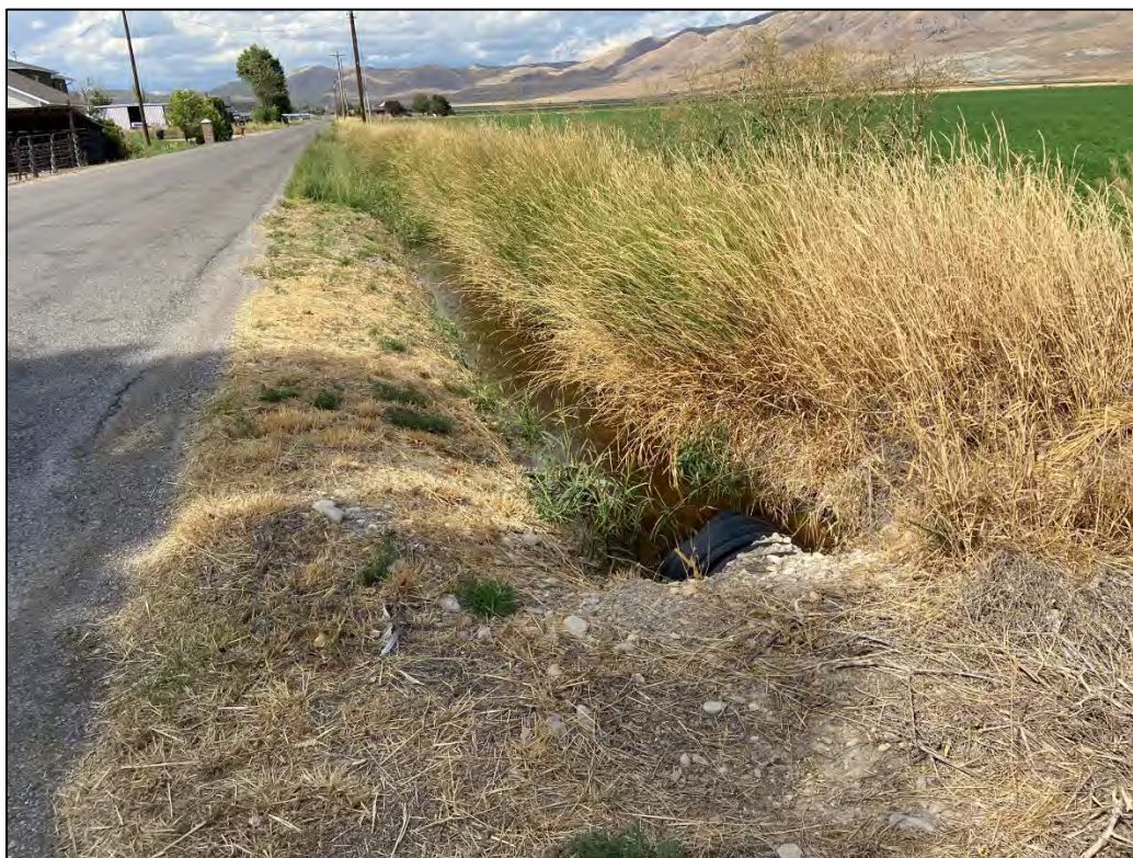
Photo 18: Looking west at a roadside ditch within the Bothwell Pocket Area.
