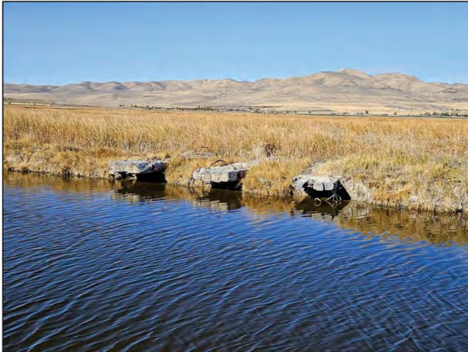
Figure 9. IF-02, isolate overview, dismantled bridge; view facing west.
