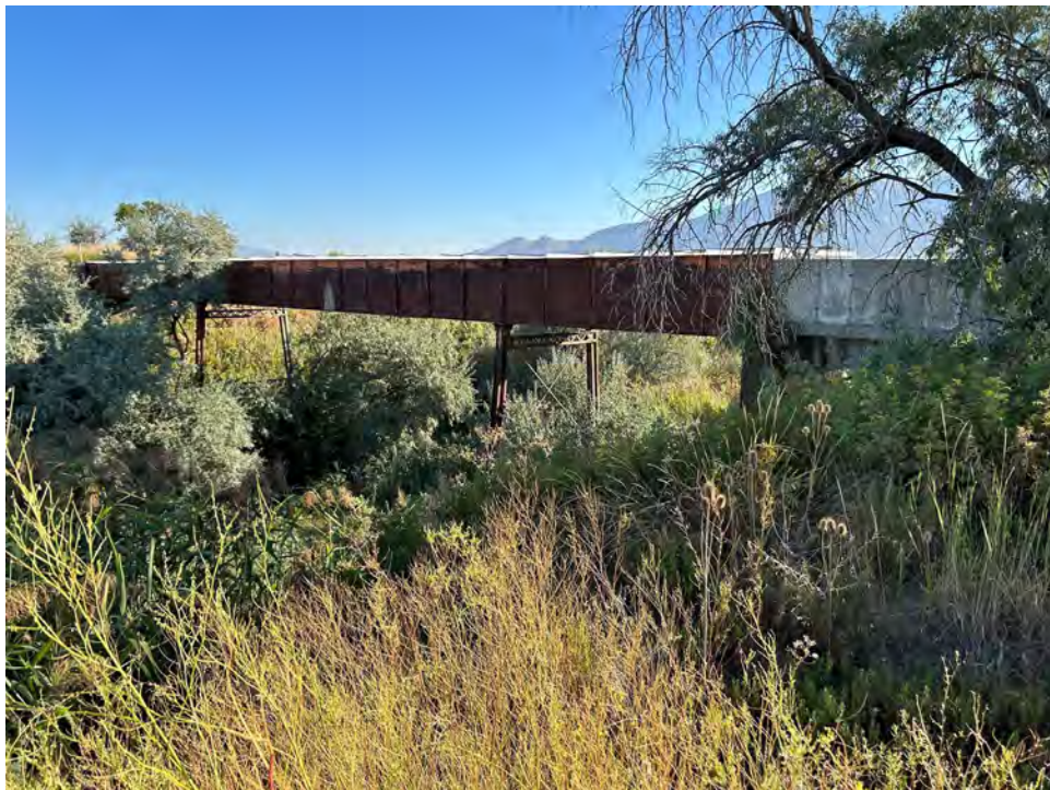
Photo 4: Canal 2 Flowing Over Bridge with Malad River Below Facing Southwest
