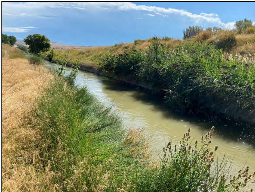
Photo 1: Dense vegetation along a concrete-lined section of the Hammond Canal in an agricultural area outside of Fielding, south of the BRCC Canyon Area.
