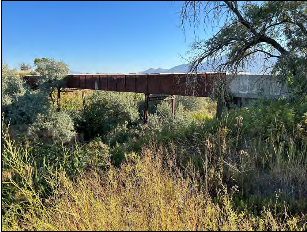
Photo 21: Looking southwest at the Red Flume Replacement Location.
