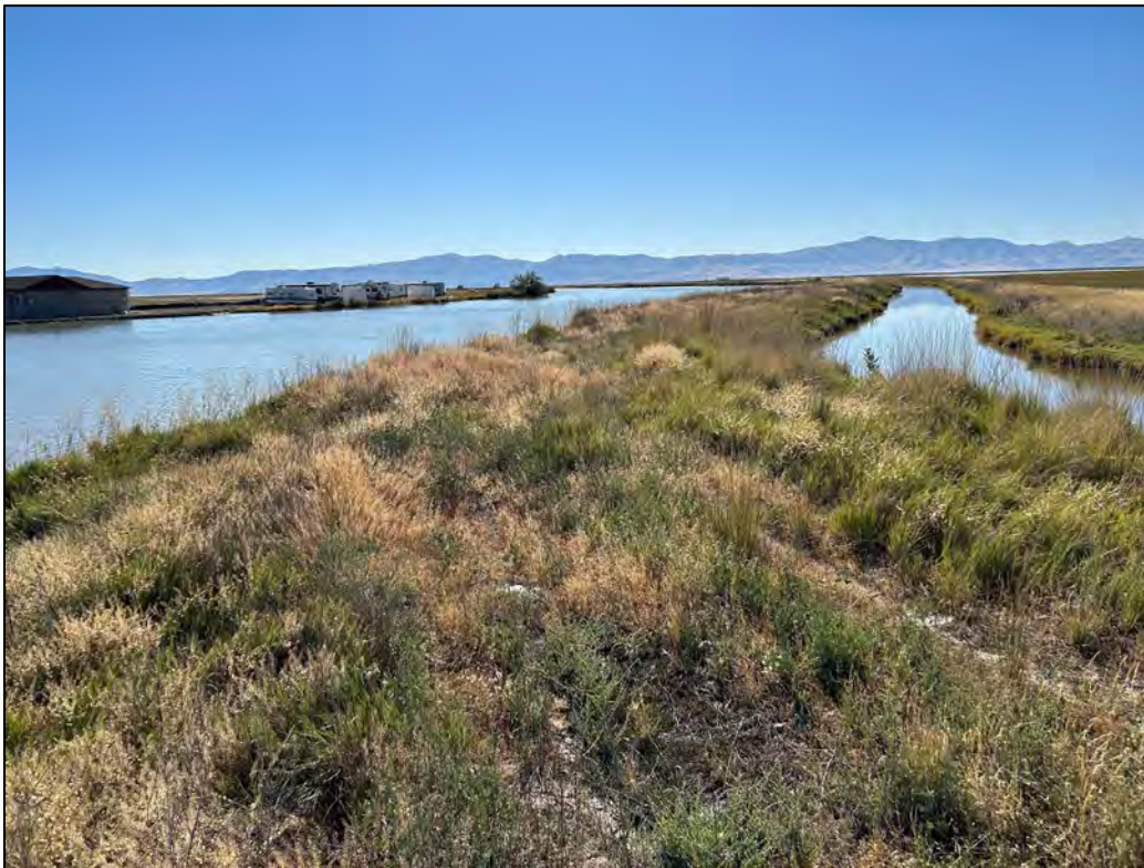
Photo 24: Looking west at the Bear River Duck Club Area.
