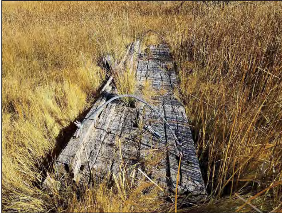
Figure 8. IF-01, isolate overview, dismantled bridge; view facing northeast.
