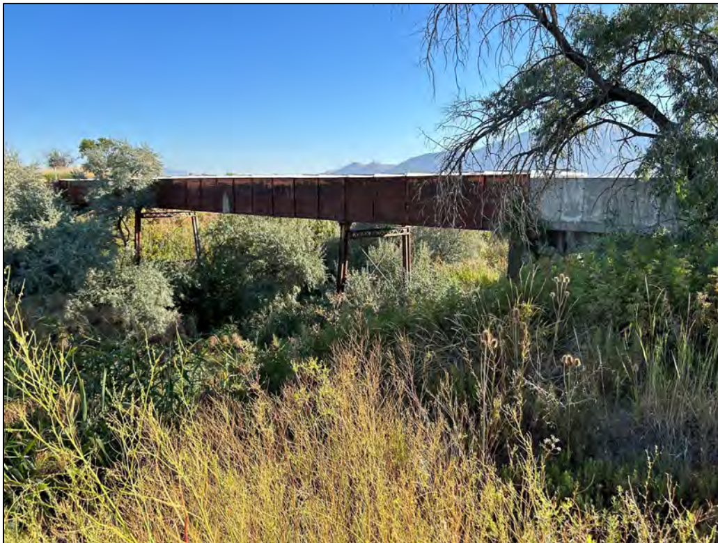
Photo 26: Looking southwest at the Red Flume Replacement Location.
