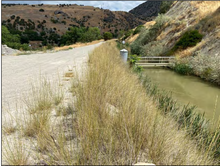
Photo 7: Lined portion of the Hammond Canal in the canyon area, looking northwest towards the dam.
