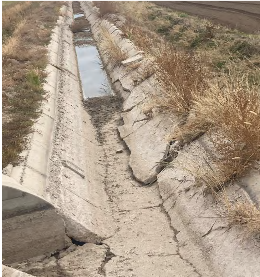
Figure 2.1.4.1. Highland Ditch existing conditions.
