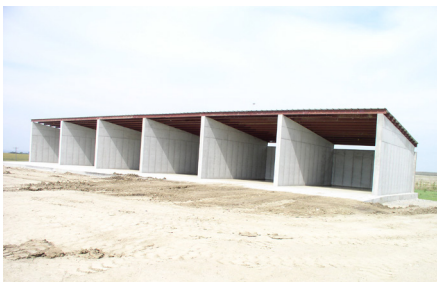
Static Pile, Concrete Bins
